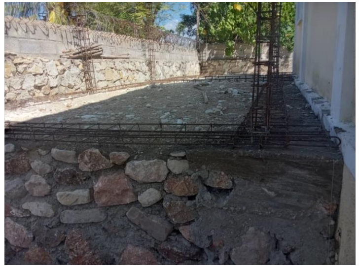
December 05, 2021, new restrooms beside church.
